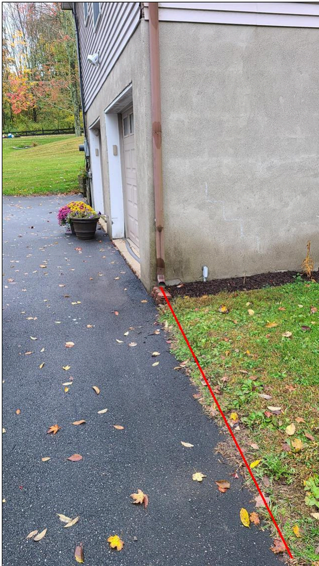
C. Item 1(Picture) Rear downspout
