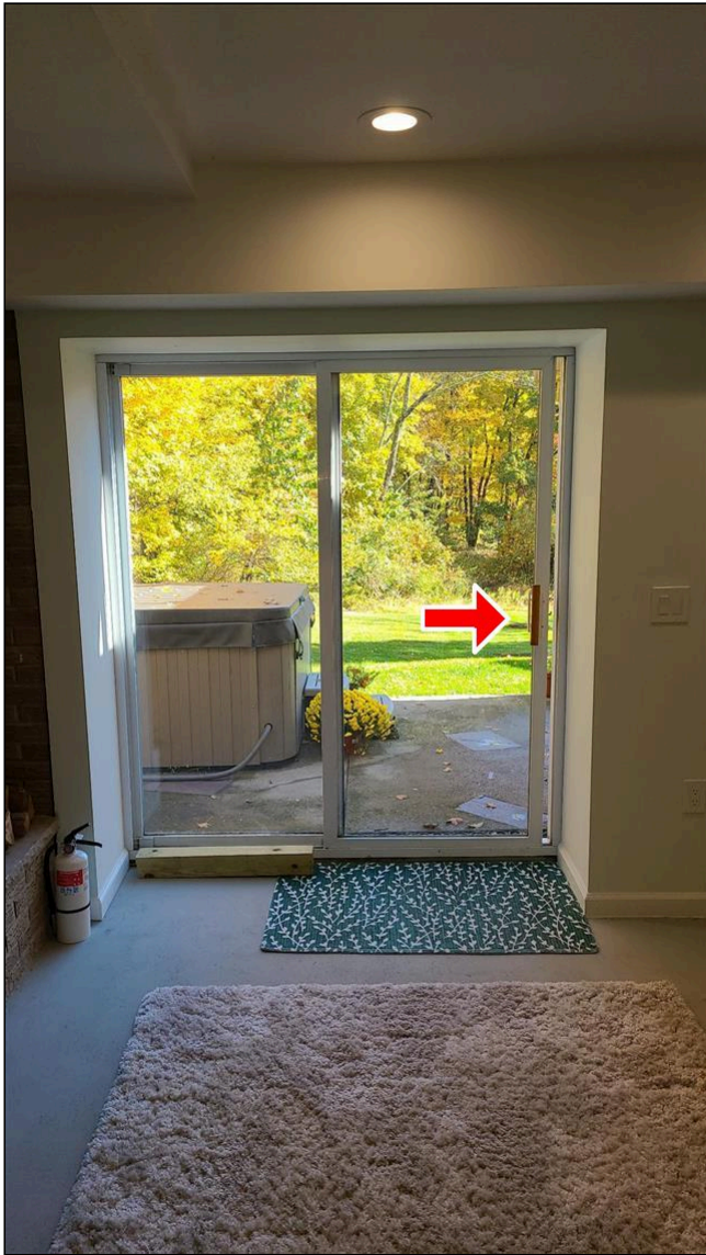
H. Item 9(Picture) Basement slider
