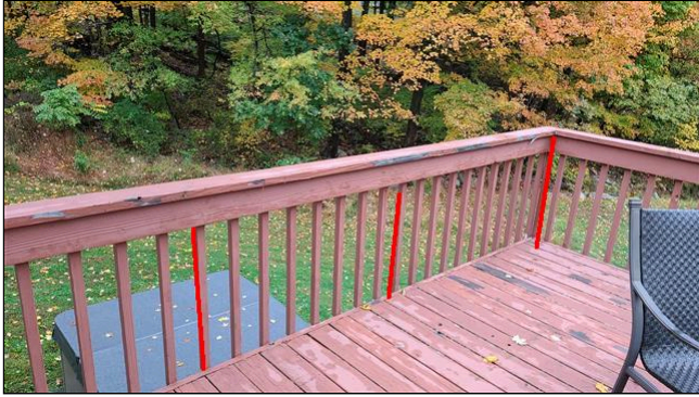
K. Item 1(Picture) Deck railing
