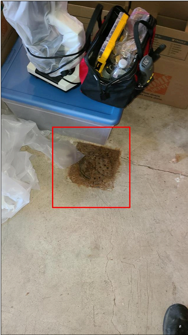
B. Item 5(Picture) Garage drain
