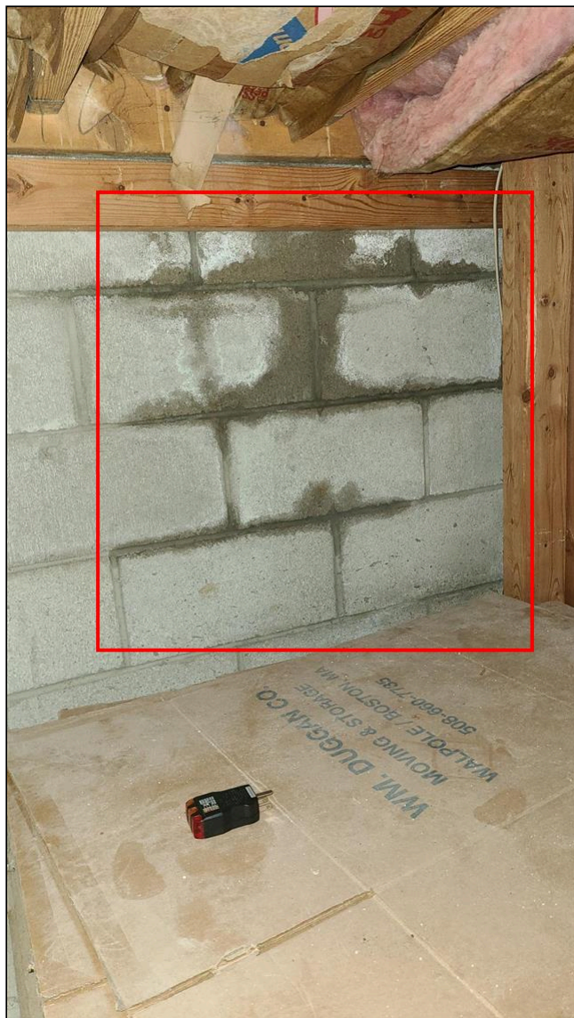
A. Item 1(Picture) Crawlspace
