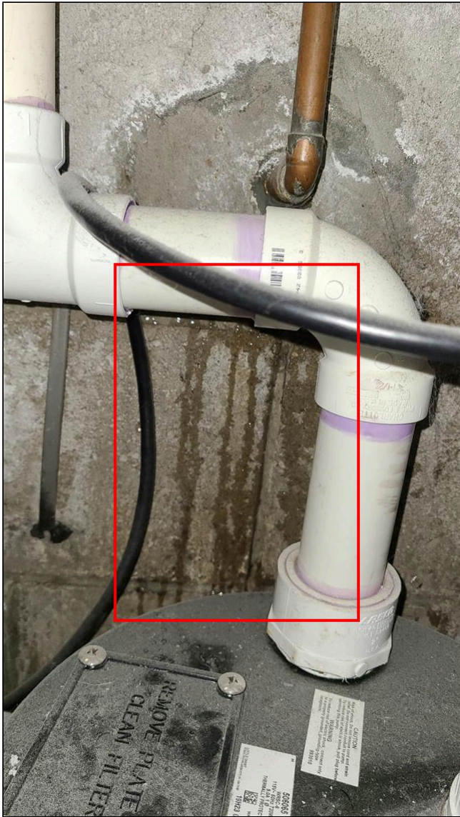
A. Item 3(Picture) Laundry room
