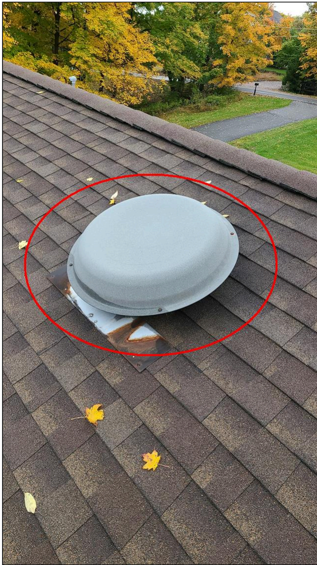
C. Item 1(Picture) Attic vent cover
