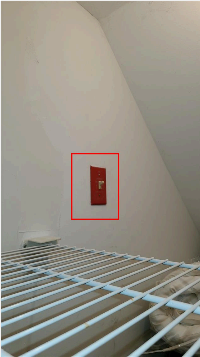
B. Item 3(Picture) Furnace emergency shut-off
