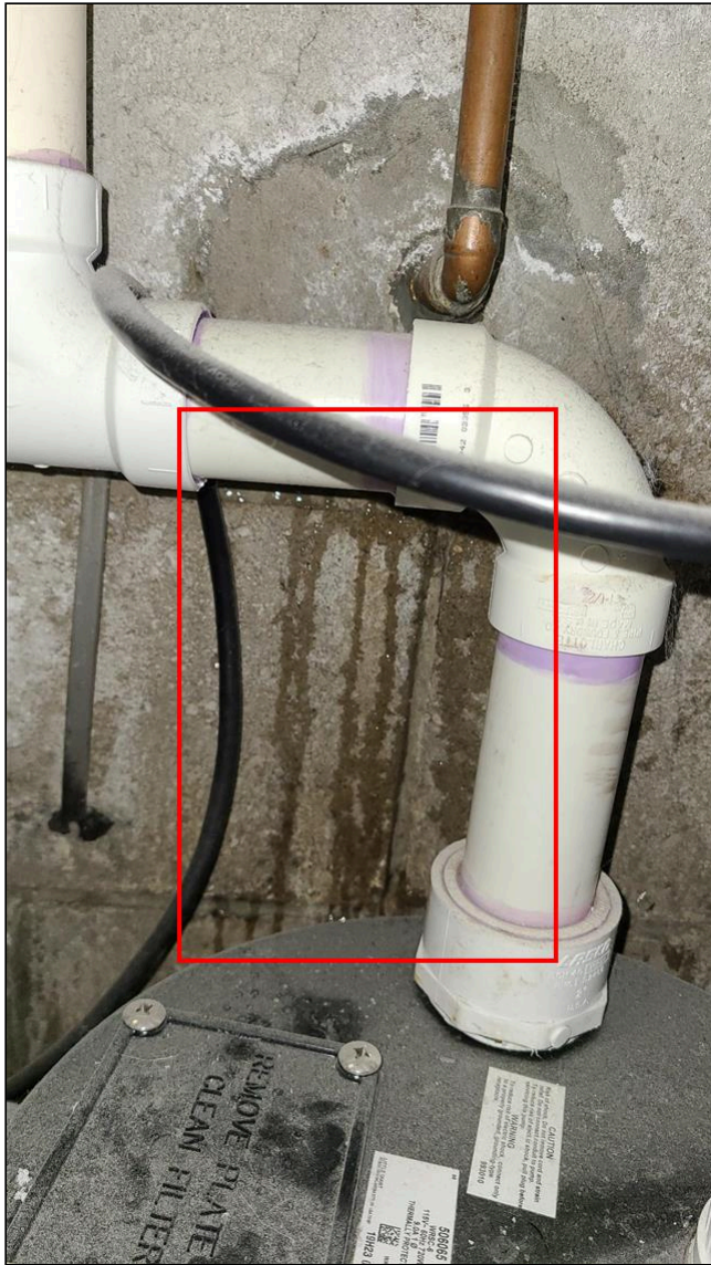
A. Item 3(Picture) Laundry room
