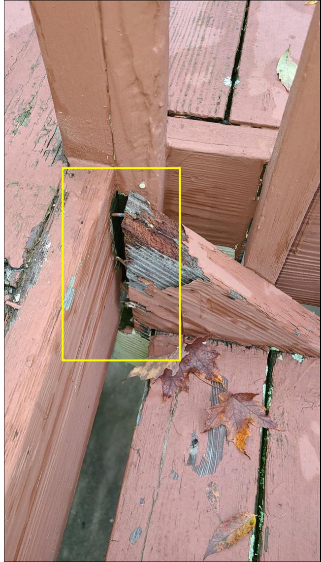
K. Item 2(Picture) Stairs
