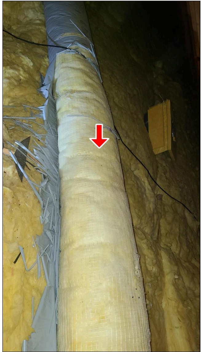
C. Item 6(Picture) Attic
