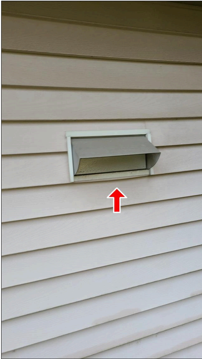
C. Item 5(Picture) Kitchen Microwave vent
