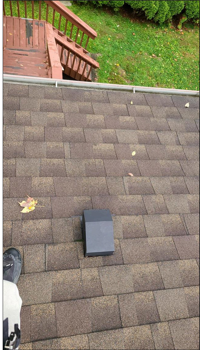
C. Item 4(Picture) Roof vent
