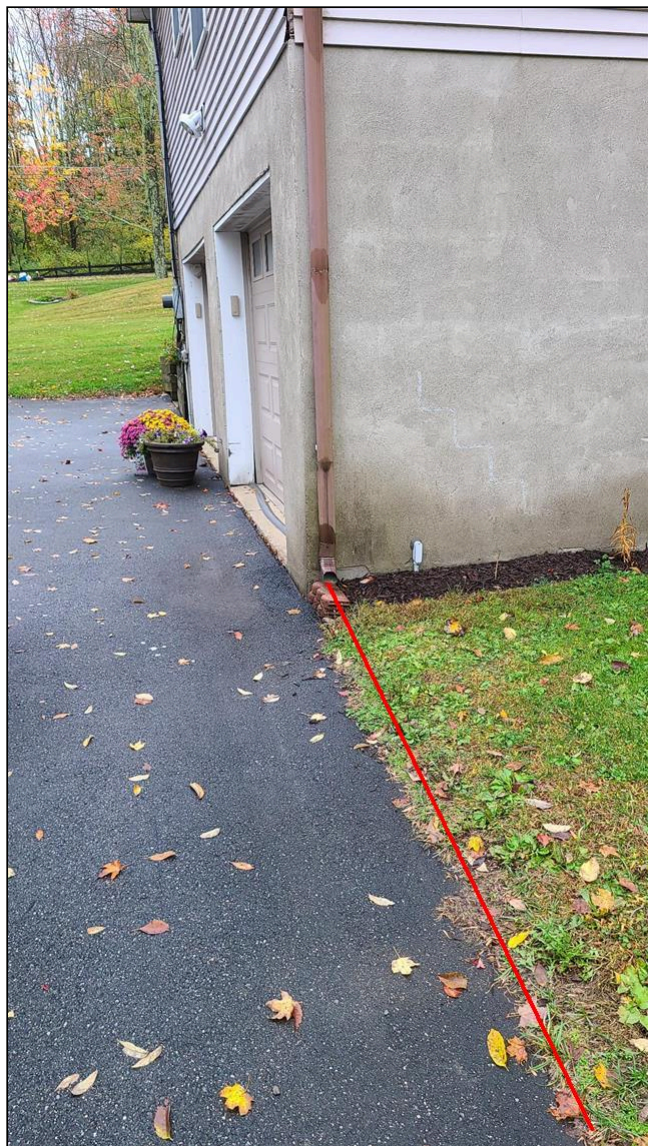
C. Item 1(Picture) Rear downspout
