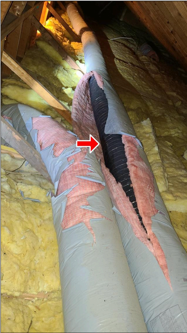
C. Item 7(Picture) Attic
