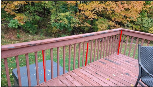
K. Item 1(Picture) Deck railing
