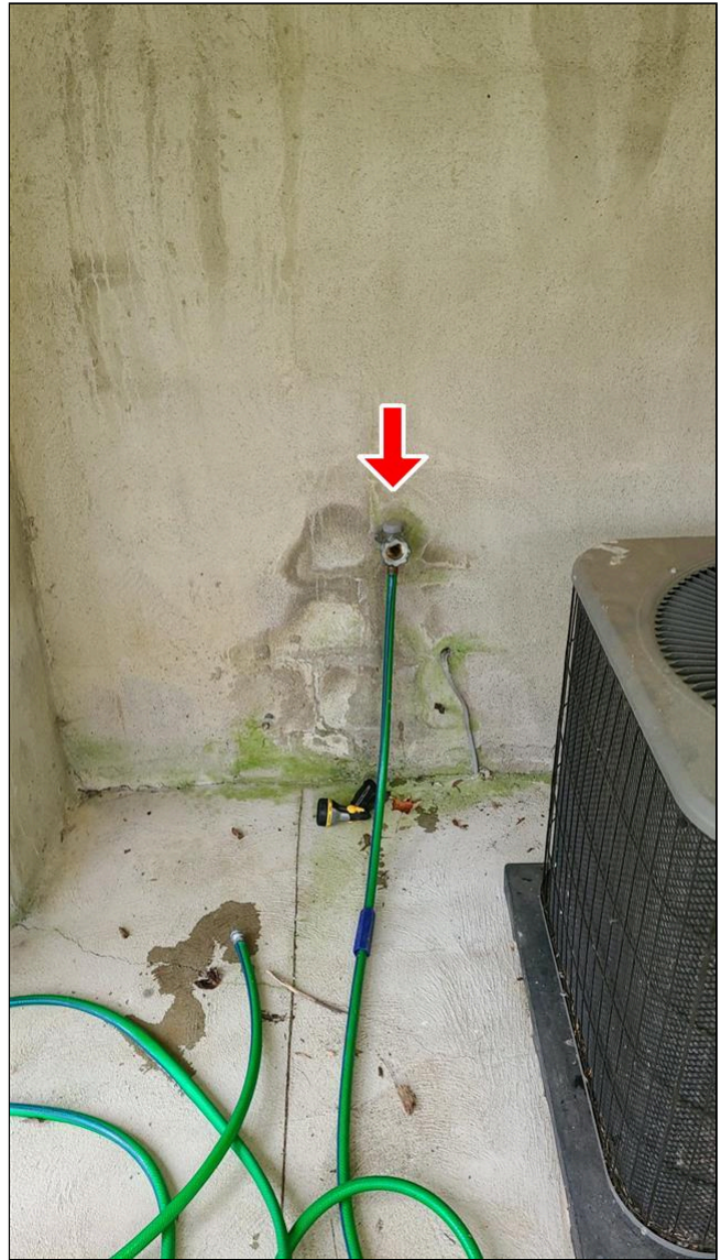
A. Item 2(Picture) Rear of the home
