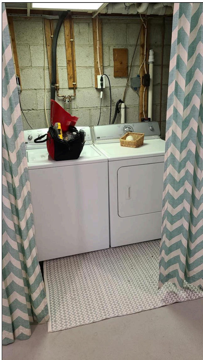
M. Item 1(Picture) Washer and dryer were working when tested.
