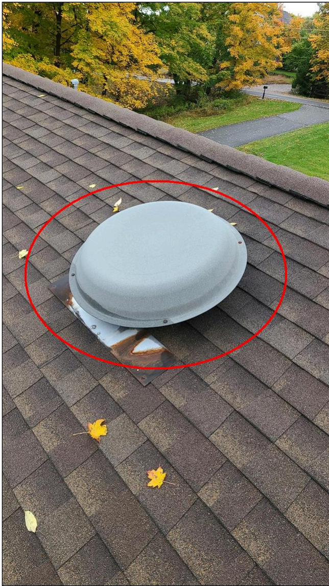
C. Item 1(Picture) Attic vent cover
