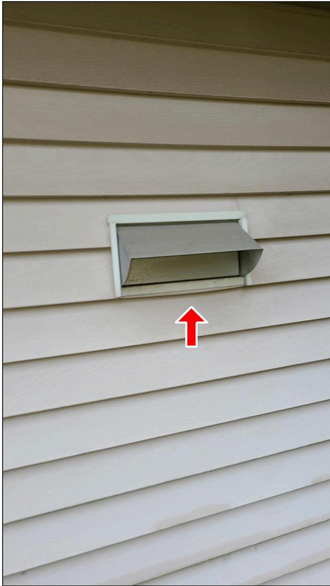
C. Item 5(Picture) Kitchen Microwave vent
