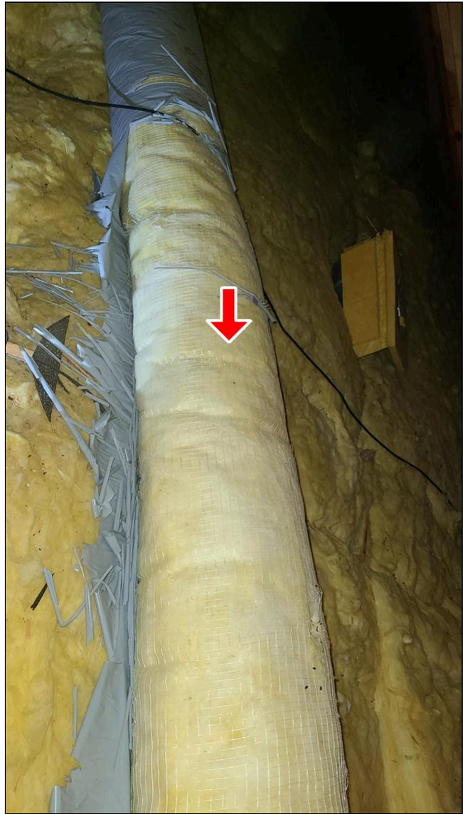
C. Item 6(Picture) Attic
