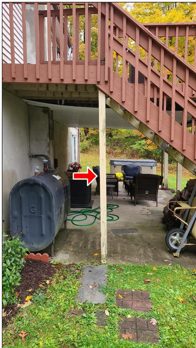
K. Item 3(Picture) Stair post
