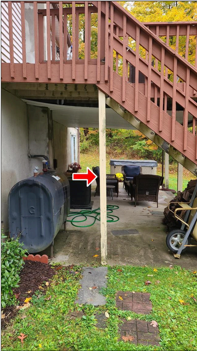
K. Item 3(Picture) Stair post
