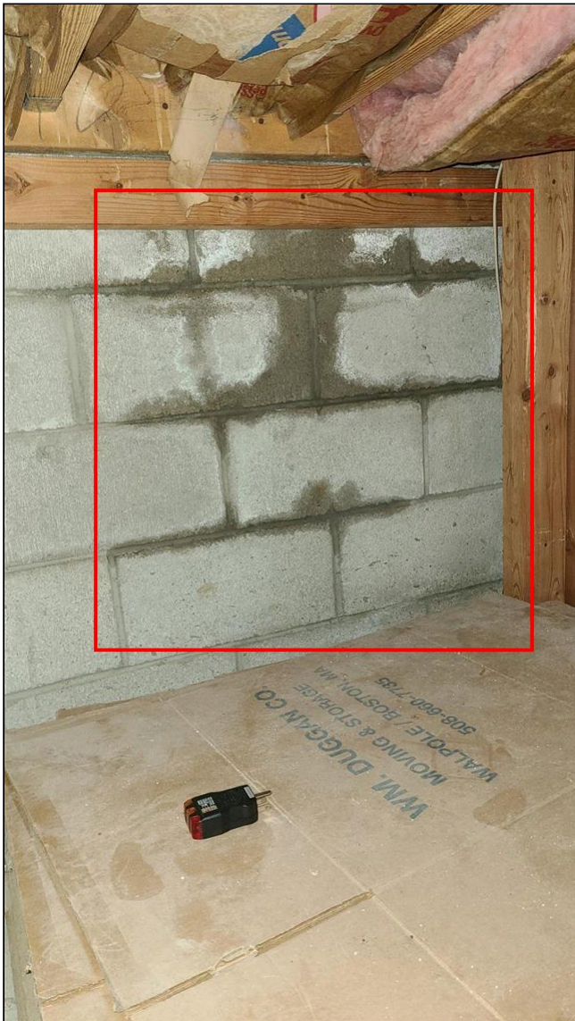
A. Item 1(Picture) Crawlspace
