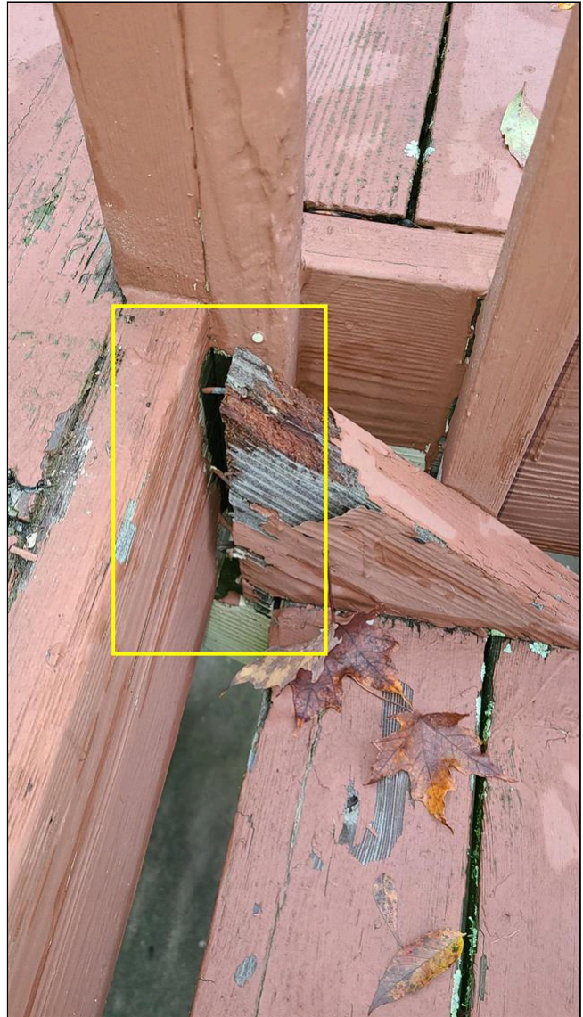
K. Item 2(Picture) Stairs
