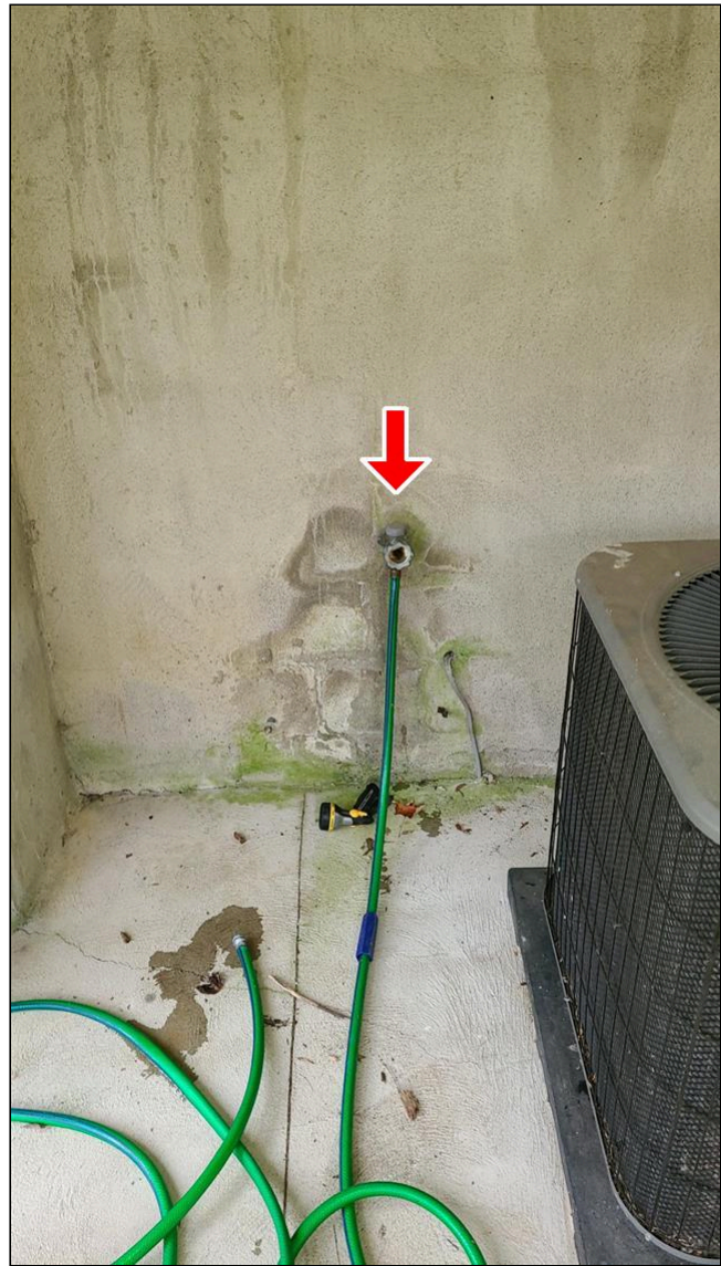
A. Item 2(Picture) Rear of the home
